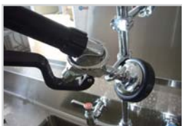
Pre-Rinse Faucet and Sink
